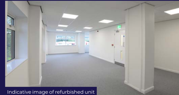
Indicative image of refurbished unit
